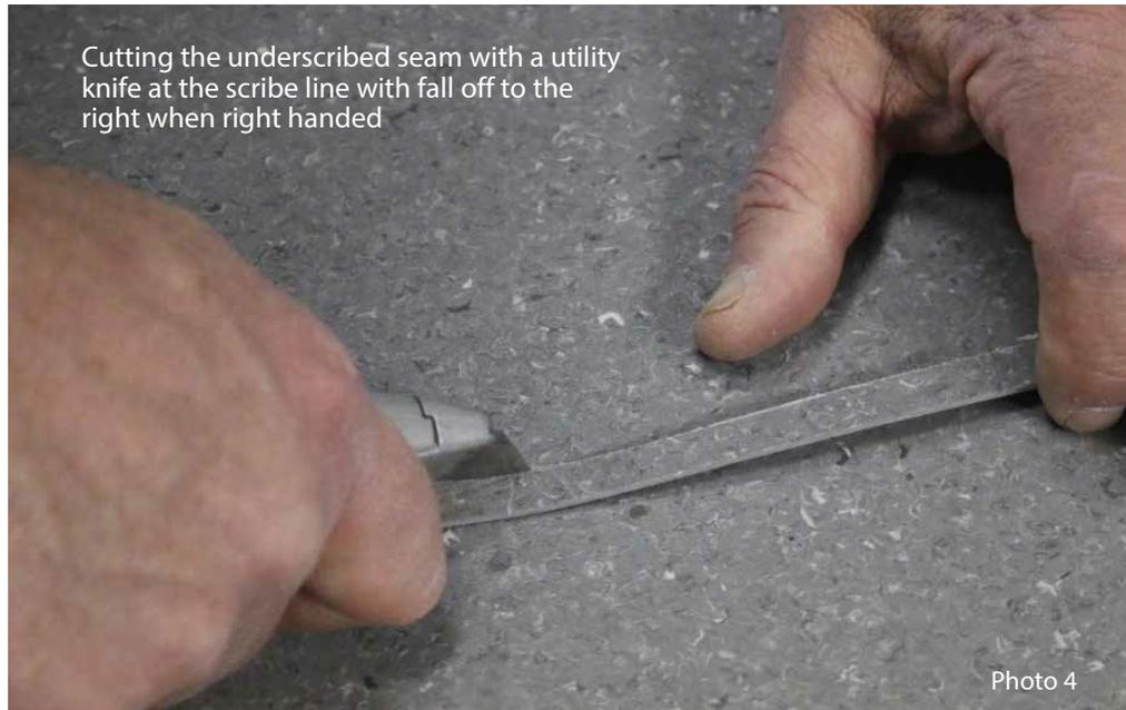
4. Once you have completed the scribing and cutting of the seam (*see net fit in Photo 5*), roll the seam area with a steel hand seam roller. Roll diagonally across the seam six inches on both sides. This technique minimizes the risk of pushing adhesive into the seam and contaminating. Once you have scribed, cut and hand rolled the seam, then roll the entire area again in two directions with 75-100 lbs. 3-section roller.
