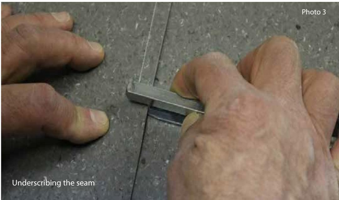
3. Cut the seam using a utility knife (straight or hook blade). Cut the seam by following the scribe mark Your fall off should be to your right if you are right handed and to your left if you are left handed. (*see Photo 4*)
